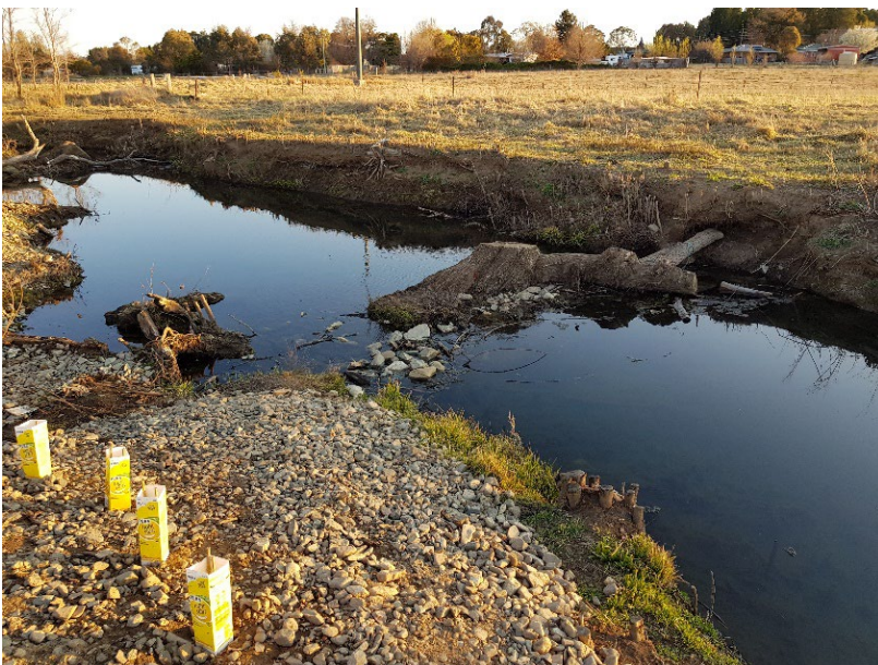
Photo 9 – “Riffle” zone being crfeated in Dumaresq Creek
